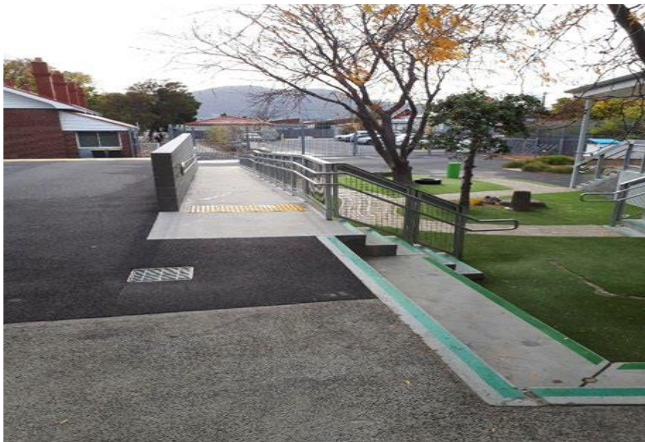
Figure 3: Area at the top of the concrete ramp with the sunken sitting area depicted to the right of the photograph.
