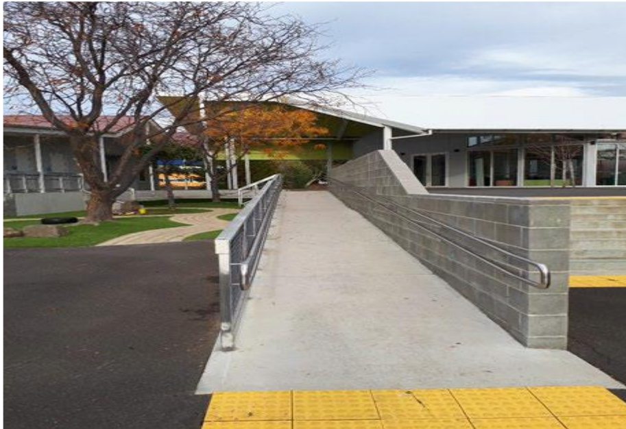
Figure 2: Concrete ramp leading to sunken sitting area.
