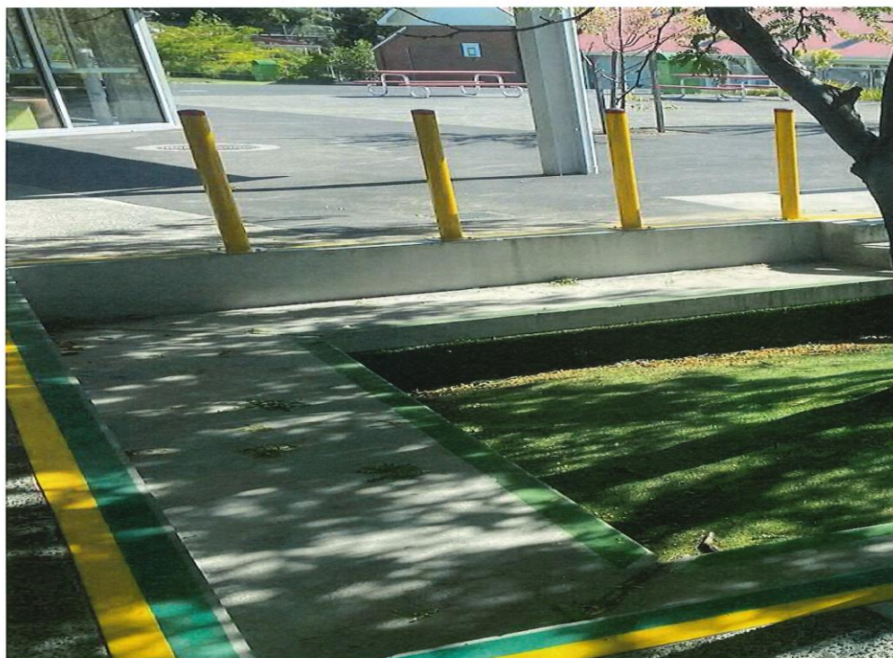
Figure 6: Permanent bollards installed in compliance with the Improvement Notice.
