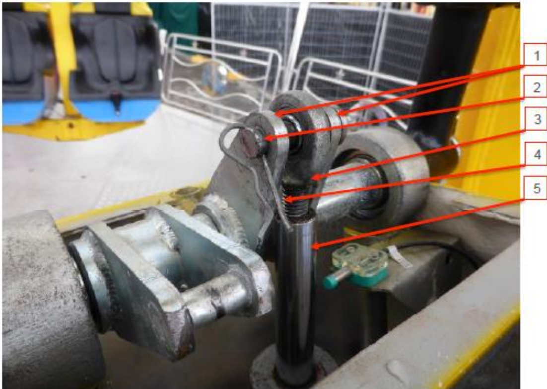
Figure 34 Airmaxx 360 Arm 6 RHS (seat 11) primary lock cylinder connection (P1010540.JPG)
